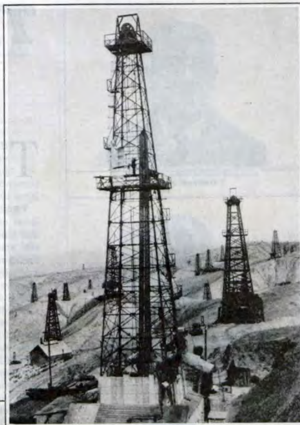
The Steel Derrick of the Standard Oil Company of California in Use at the Mascot No. 1 Well
