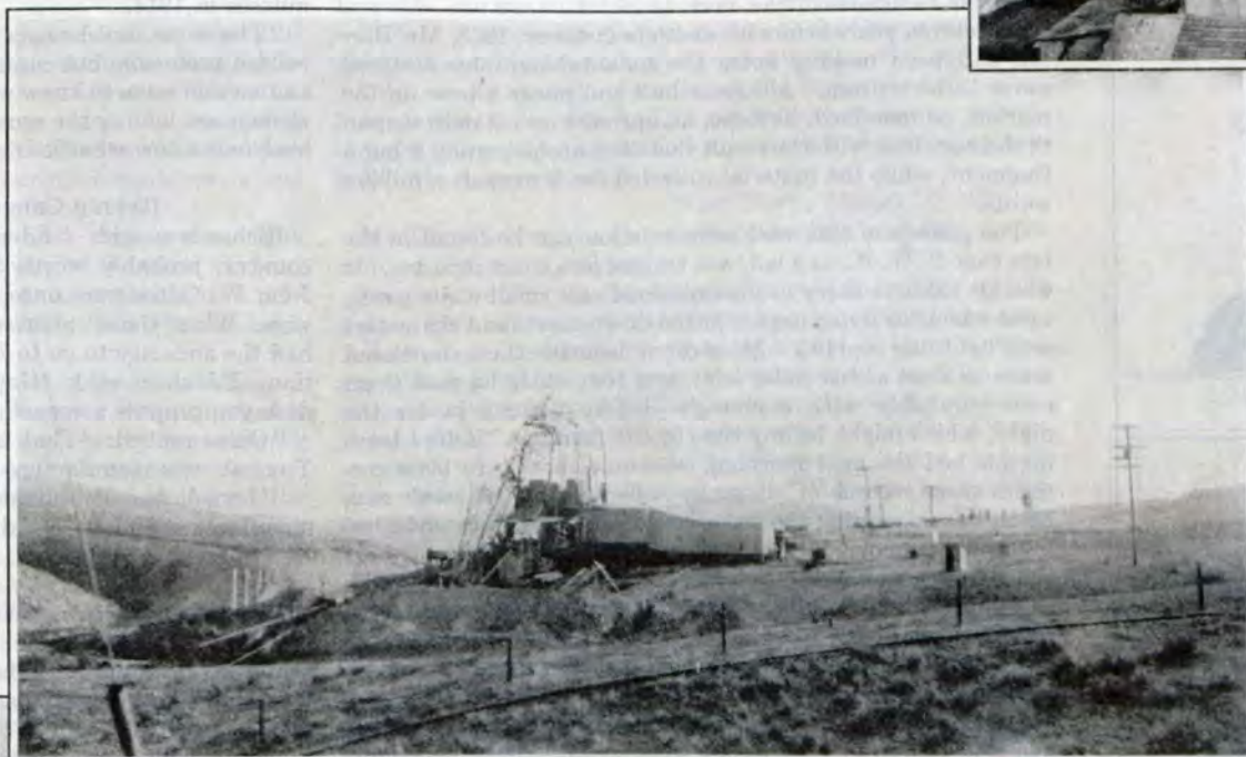
A Blow-Out in a Marland Well at Kettleman Hills, Showing Enormous Power of Gas Which Twisted the Massive Steel Derrick
