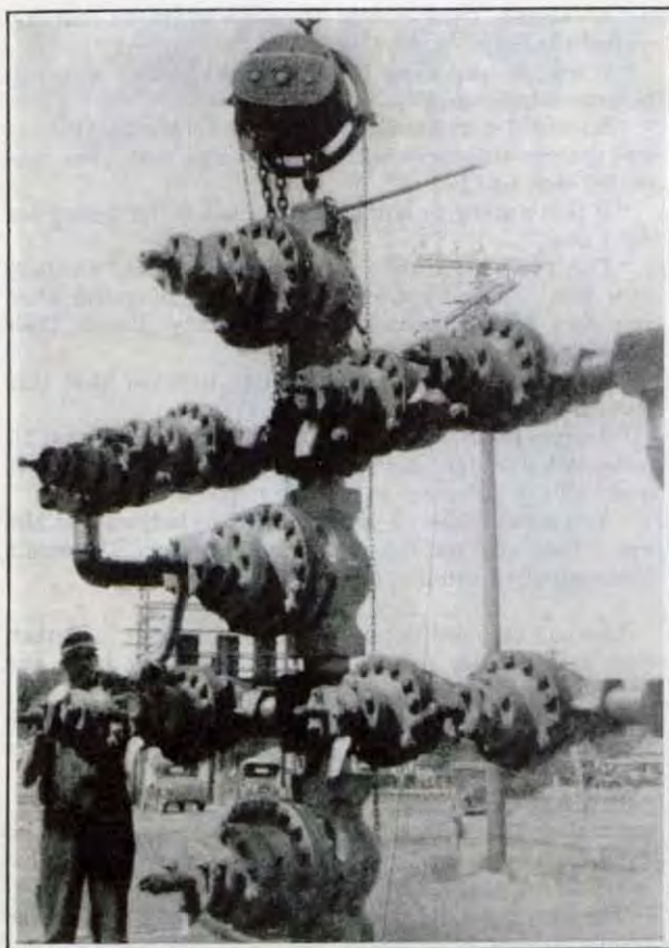
An Assembly of Gates and Valves for the Control of Enormous Gas Pressure at the Kettleman Hills Field
