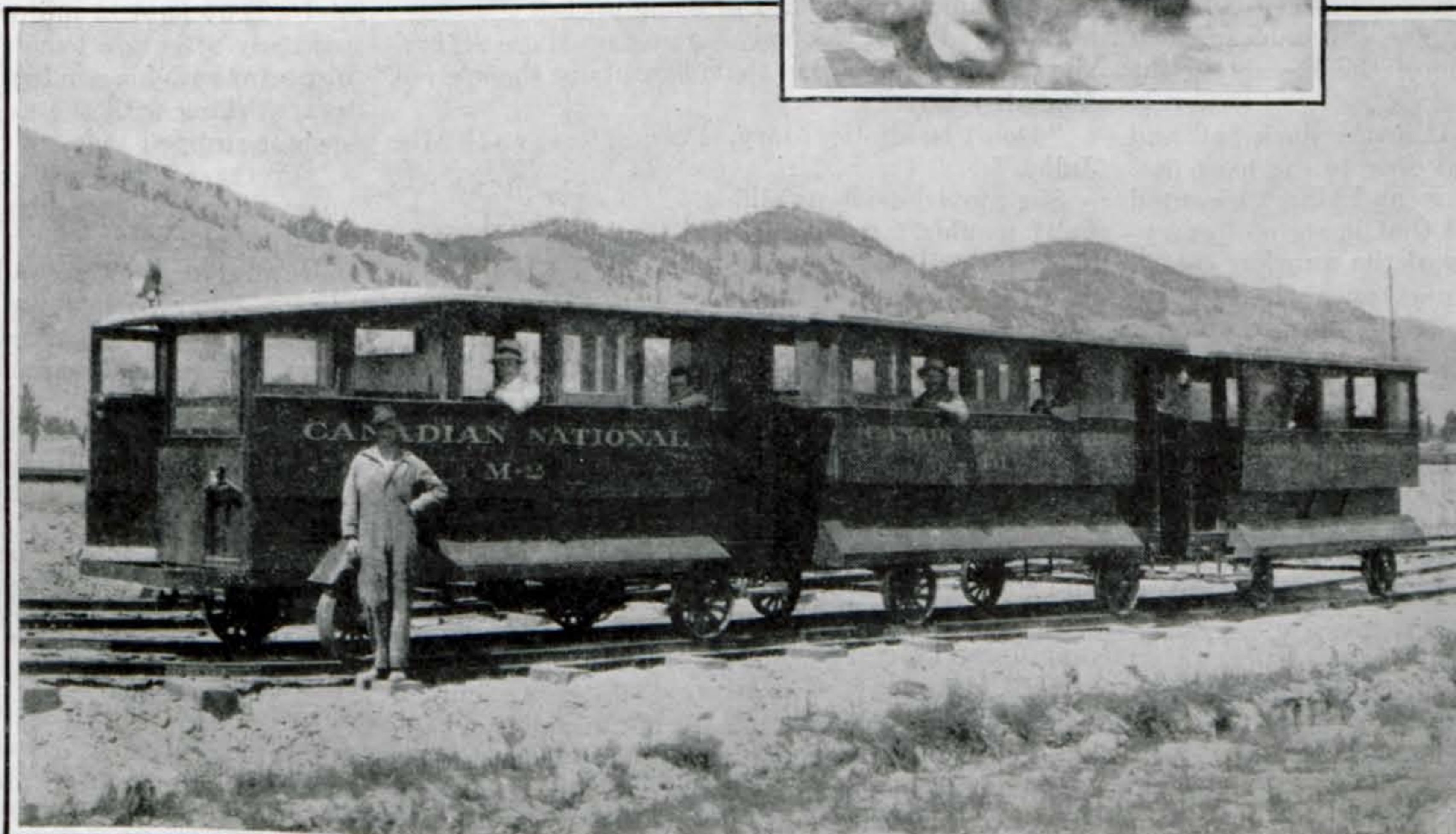
This "Train" is Powered by Nothing More Than an Automobile Engine
